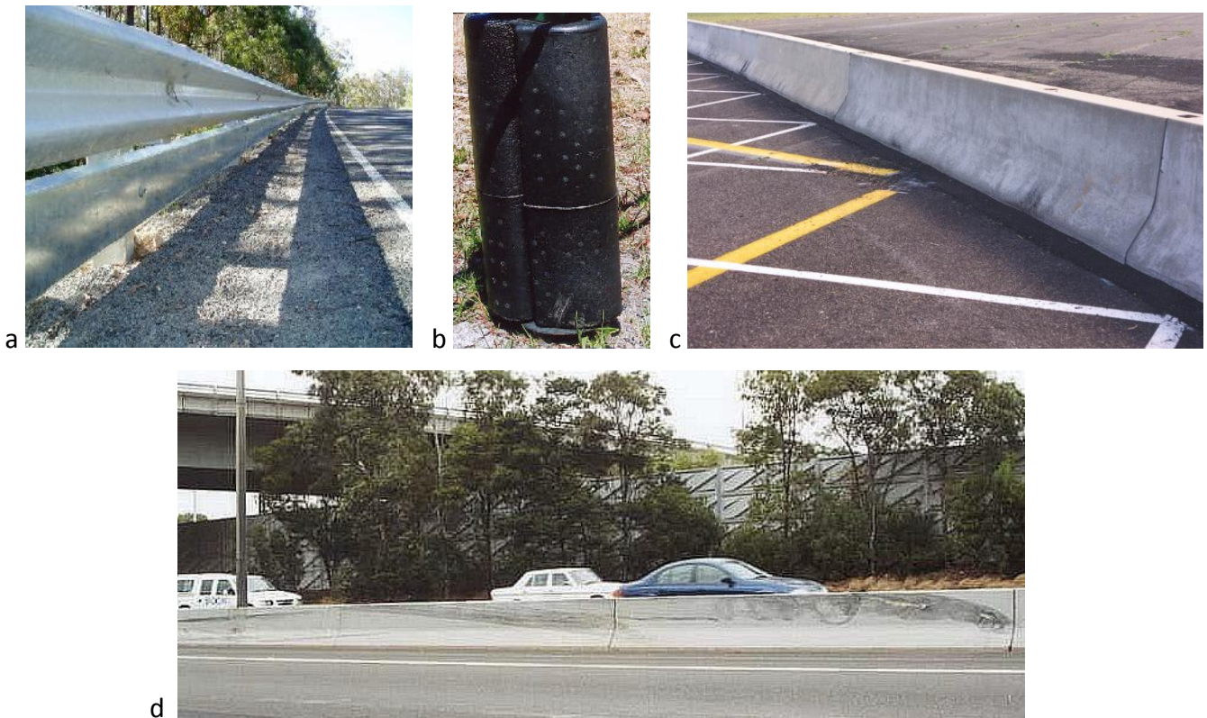
Figure 1: Examples of; a) steel rub-rail system, b) padded post protector and c) continuous concrete barrier d) wheel prints on concrete barrier showing evidence of vehicle launching
