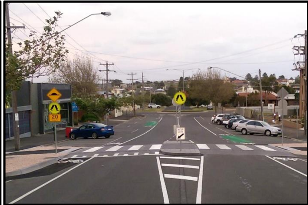
Koroit Street, Warrnambool
