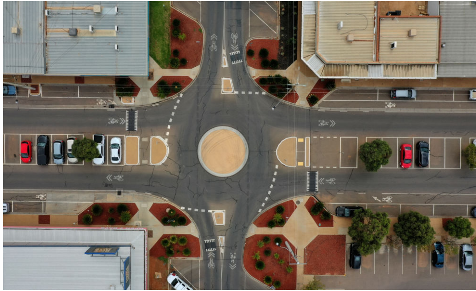
Figure 1: Low Cost Implanted Compact Roundabout
