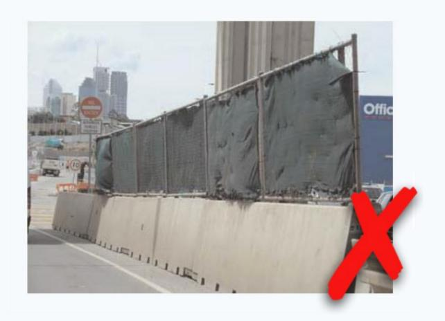
Temporary fence panels mounted on PCBs. Horizontal rails constitute a potential spearing hazard and are not permitted.
