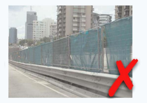
Temporary fence panels mounted on a steel barrier system. It is unlikely that the method of mounting is approved by the barrier manufacturer and could compromise the barrier performance. Horizontal rails constitute a potential spearing hazard and are not permitted.
